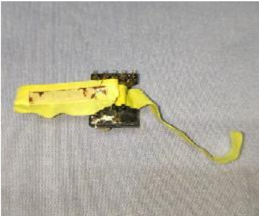
Picture 24 Transformer view
